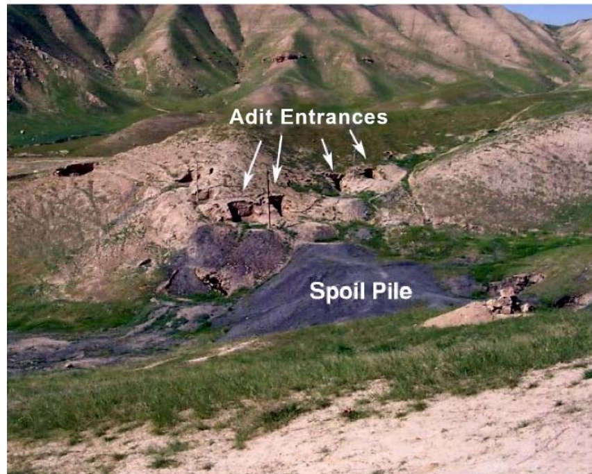
Figure 7. Hand-dug adits for manual coal extraction (after SanFilipo 2005).
