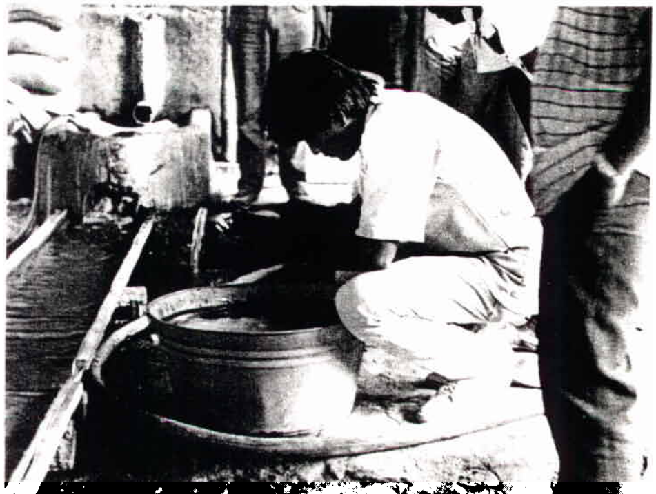
3. Gravity separation and recovery system using fabric lined trough and pan.
