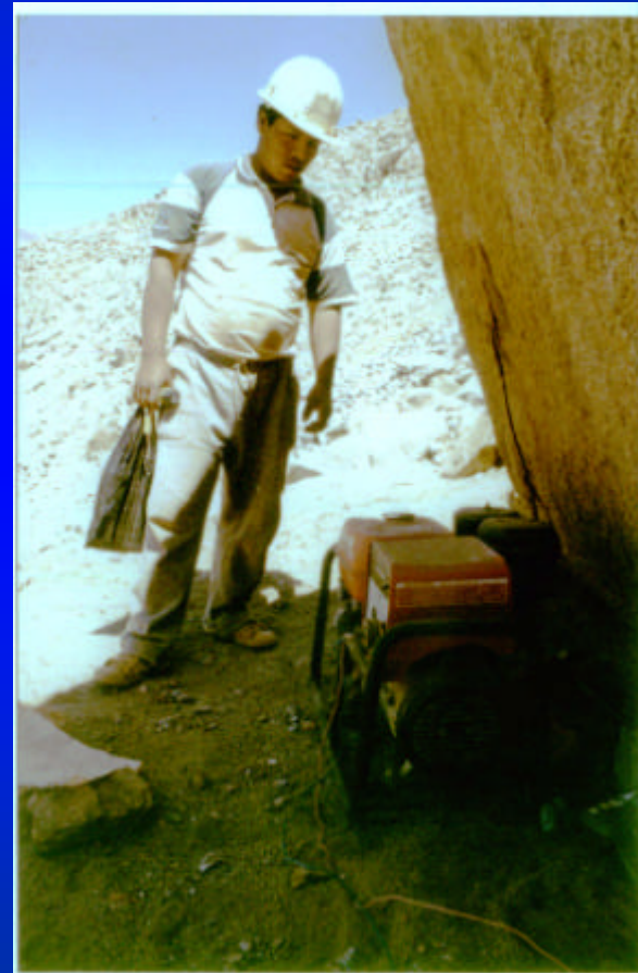
Electrical drilling machine and small generator
