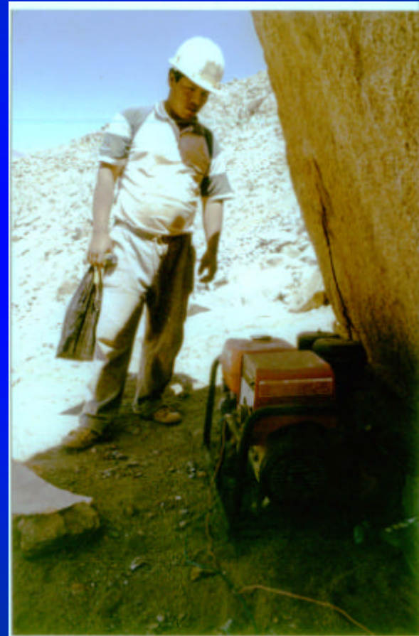
Electrical drilling machine and small generator
