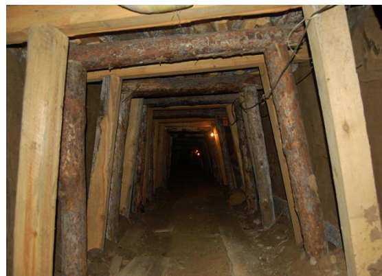
The supported mine entrance Courtesy of J. Hinton, 2007
