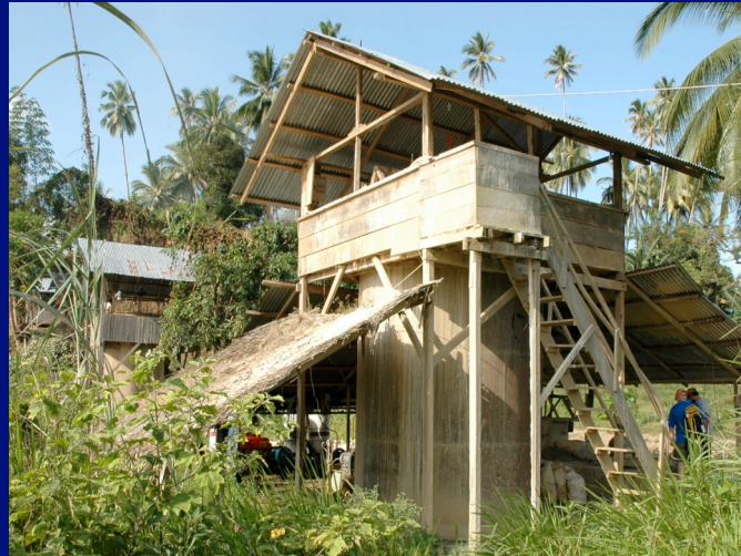
Tank Leach Sulawesi 2006
