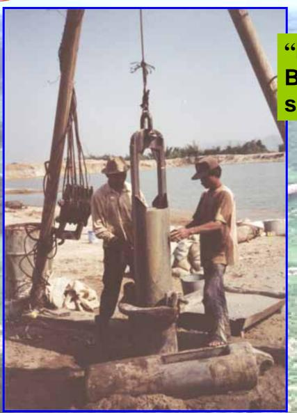
"Bore-Pile Drilling" method Bailing gravel bed layer by sand bailer.
