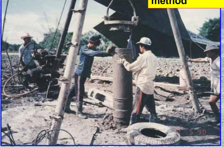
The casing can be screwed together by coupling with the used of a cable wound round the casing and pulled in by the air winch or pulled out if disconnection is wanted.
