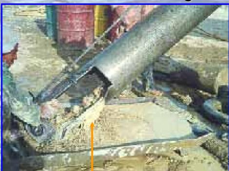
Bore-Pile Drilling - Collecting samples are ranging in size from clay particle up to boulder size of 30 cm. with bulk sample from 1-3 cu.m.
