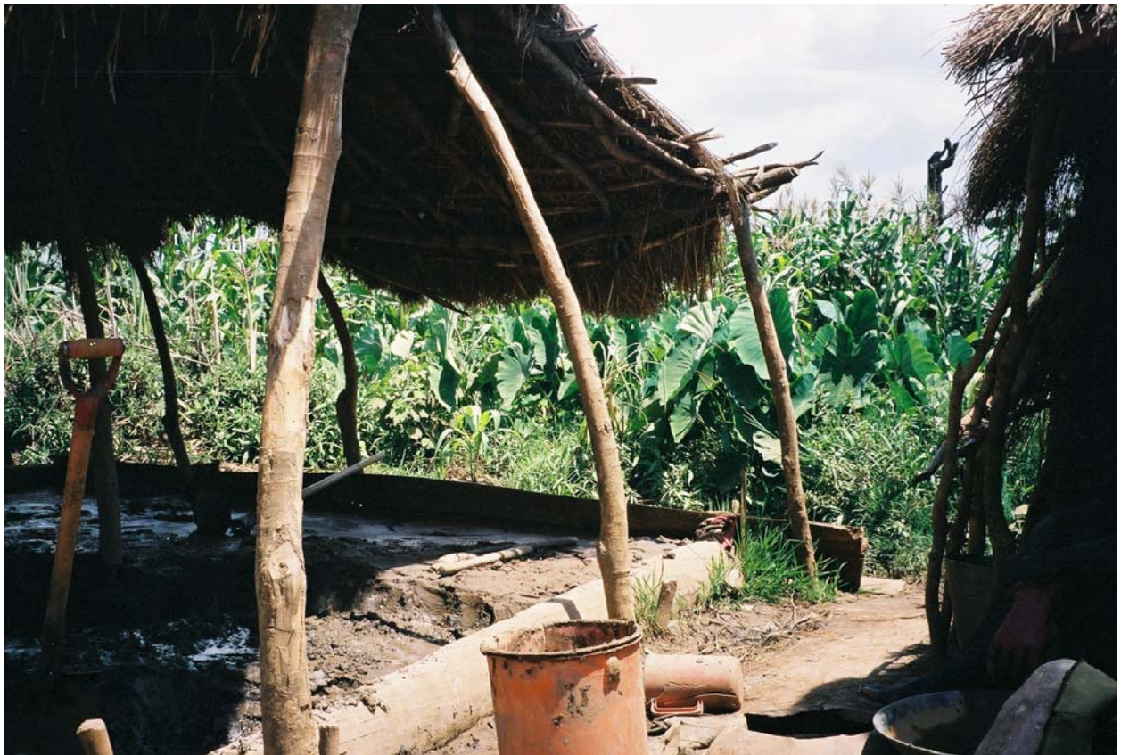
Plate 14. Wood used to retain amalgamation tailings pond at site A41-A42. Note the mercury contaminated heavy mineral tailings are being removed for re-processing. Note also, proximity of amalgamation pond to cultivated area where yams, maize and beans are being grown. There was evidence at the site that water-borne tailings contaminate the cultivated area.
