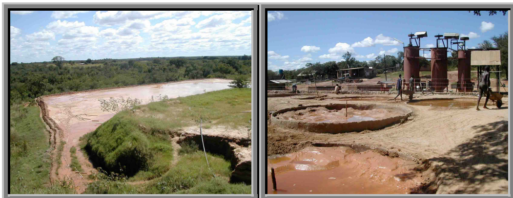
Picture 8 – Amber Rose mill: tailings and cyanidation tank.
