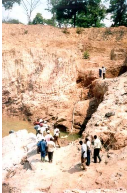
Hazards posed by highwalls and pumping of water in Ndola rural mining area
